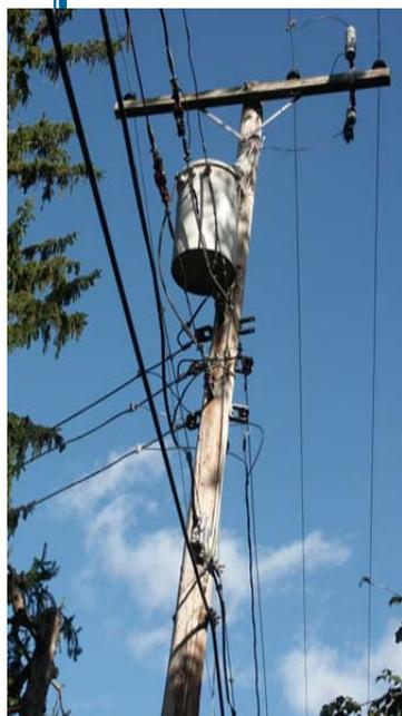
Power flows through a transformer drum on a power pole into a kilowatt-hour meter. The meter measures the amount of energy going into the home so
